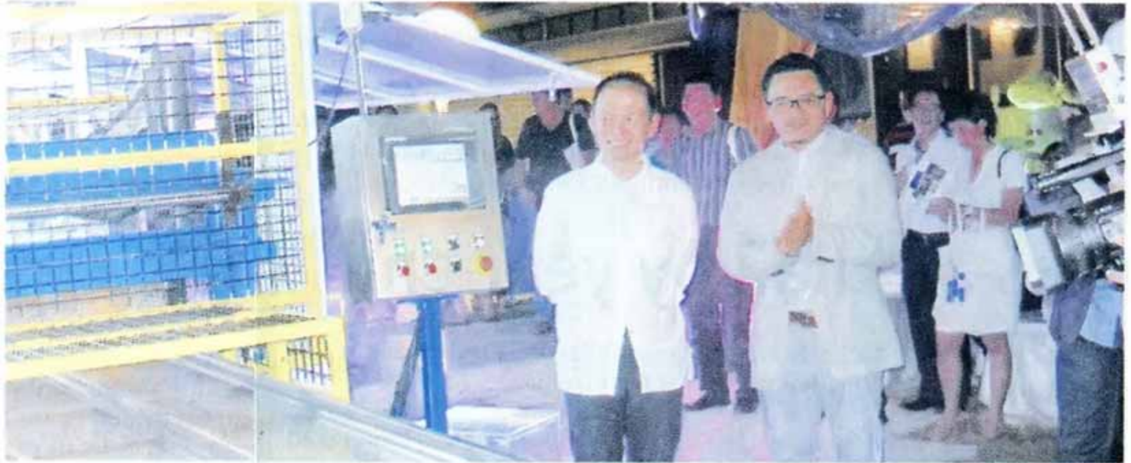
PONGSAK PADUNGKAM and Jason Tai (front right and left respectively) admiring the rolling out of Lysaght Klip-Lok Optima advanced roofing after initiating its production machine Monday.
